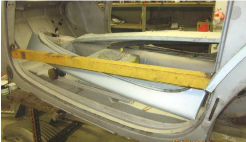
Bracing for new cill
